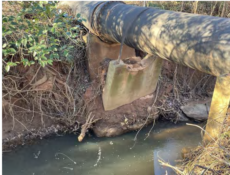
Failed Support Columns
