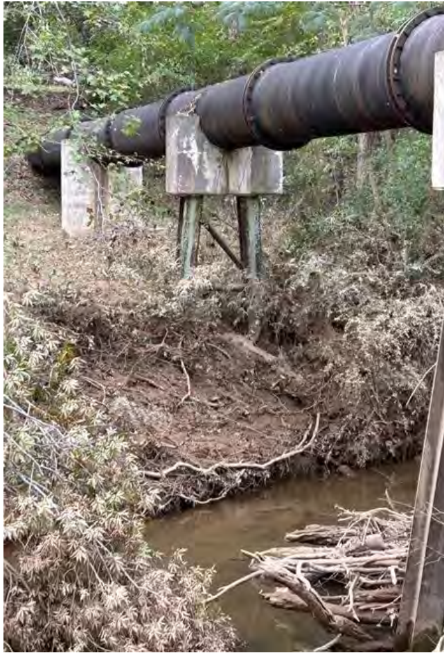
Scoured Footings on Support Pillar
