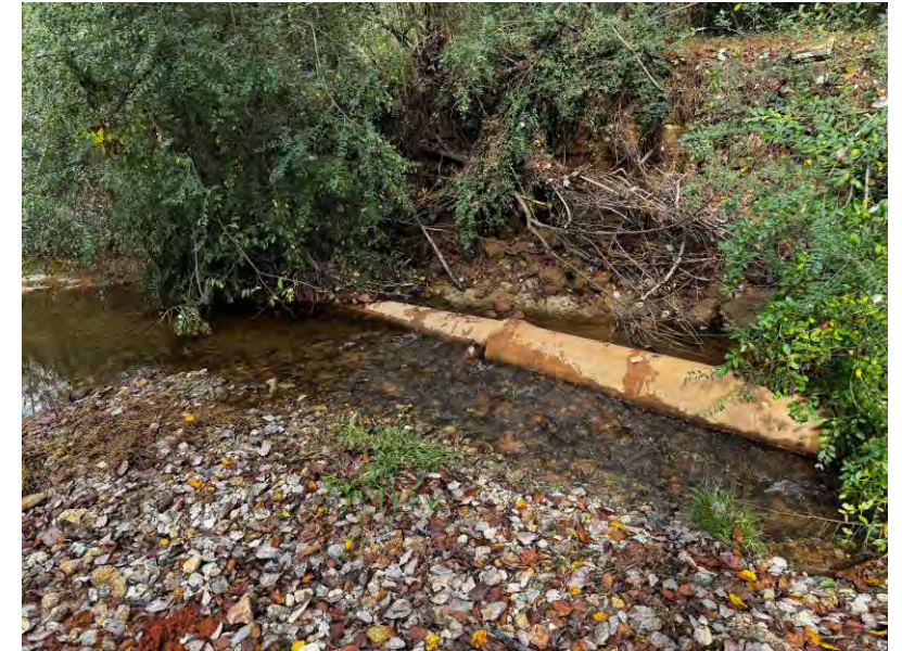
Undermining of at-grade crossings
