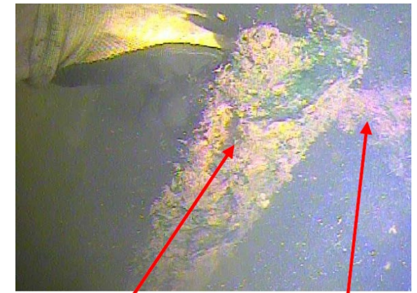
3 Wild life gate guides showing heavy corrosion. Guide off set anchors also showing heavy corrosion.
