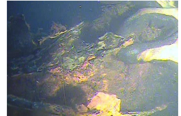
4 Corrugated steel likely used as cover/trash barrier for overflow opening. Showing extreme corrosion and section loss.
