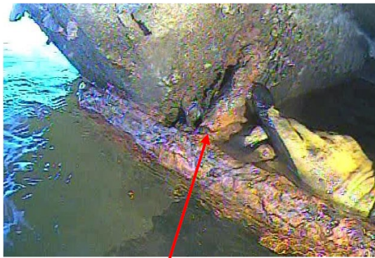
1 Horizontal angle-iron anchored to the concrete via J-Bolts. Angle-iron and J-Bolt both showing evidence of heavy corrosion.
