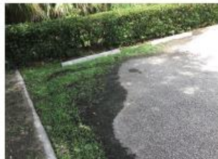
6 STANDING WATER, 12 VEGETATION (POOR) & 13 SEDIMENT (POOR)
