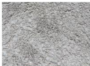
16 SMEARING (POOR)
