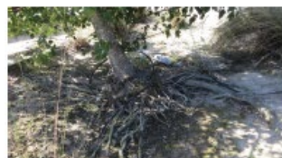
23 PLANT HEALTH (POOR - EXPOSED ROOTS AND UNSTABLE)
