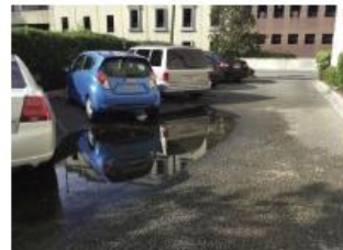
6 PONDING / STANDING WATER
