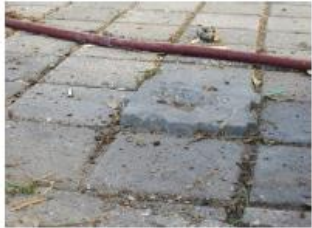
8 STRUCTURAL & 15 SEDIMENT (POOR)
