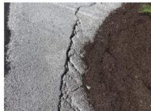
7 CRACKING-STRUCTURAL
