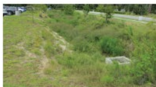
8 PRETREATMENT EROSION (SLIDE SLOPES) & 22 UNDESIRABLE VEGETATION (POOR)
