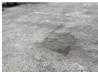
15 RAVELING (POOR)
