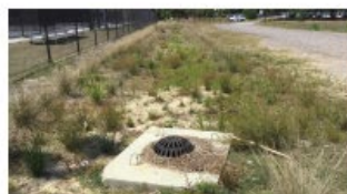
14 MULCH (NONE), 18 OUTLET DEBRIS, & 22 UNDESIRABLE VEGETATION (MARGINAL)
