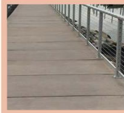
Precast Concrete Boardwalk (Permatrak, color: Savannah Brown, finish: BeachWood )
