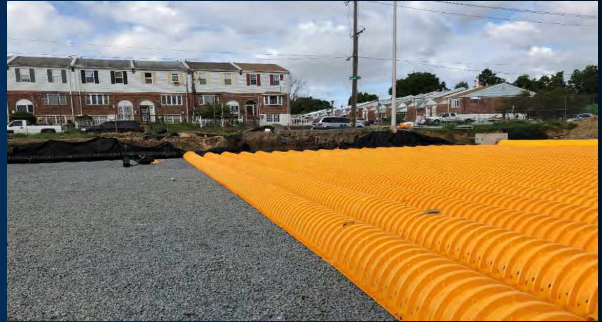
SMP 3: Construction of underground storage chambers beneath soccer field
