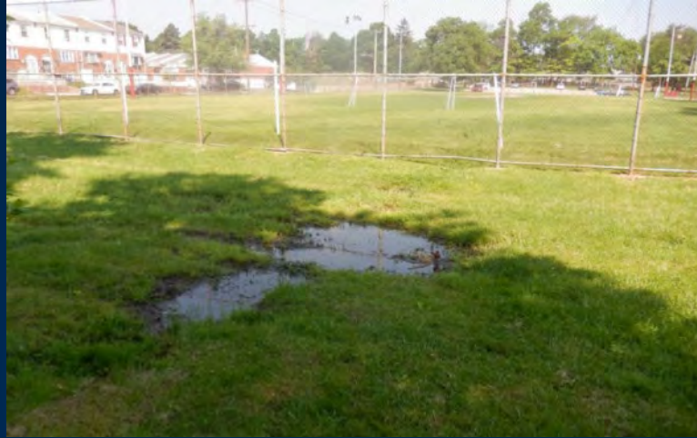
Standing water and poor drainage immediately south of the soccer field
