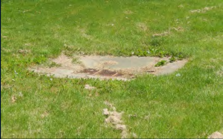
Typical yard inlet within park
