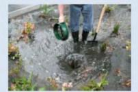
The outlet screen was filled with debris. After removal and cleaning, water can flow again
