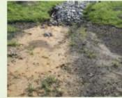
Sediment has accumulated in the infiltration area and needs to be cleaned out. Clogged media may require replacement
