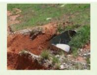
The slope near the outlet has eroded and requires repair
