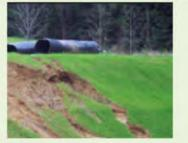
The slope of this berm has failed and eroded, requiring regrading and replanting
