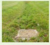
Sediment has accumulated on this inlet grate and needs to be cleaned off.
