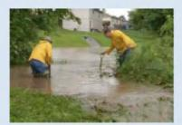
The outlet has clogged, which has led to flooding of the BMP and nearby property.
