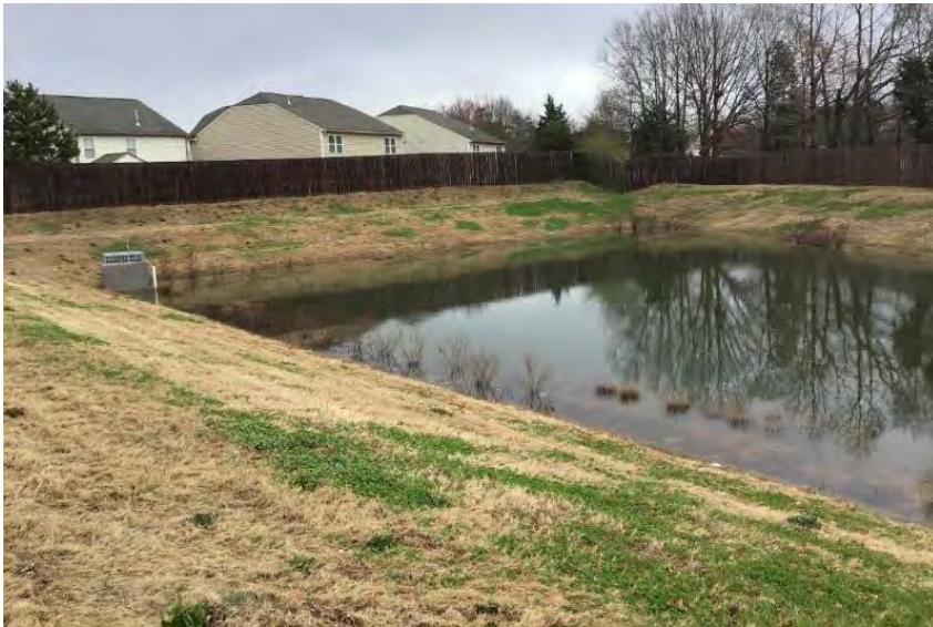
Pond is well vegetated with clean stone in spillway
