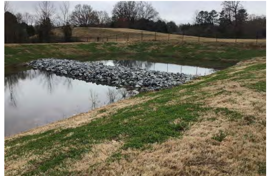
Pond is well vegetated with clean stone in spillway
