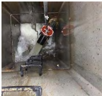
Control structure is clean, functioning properly, and exercised
